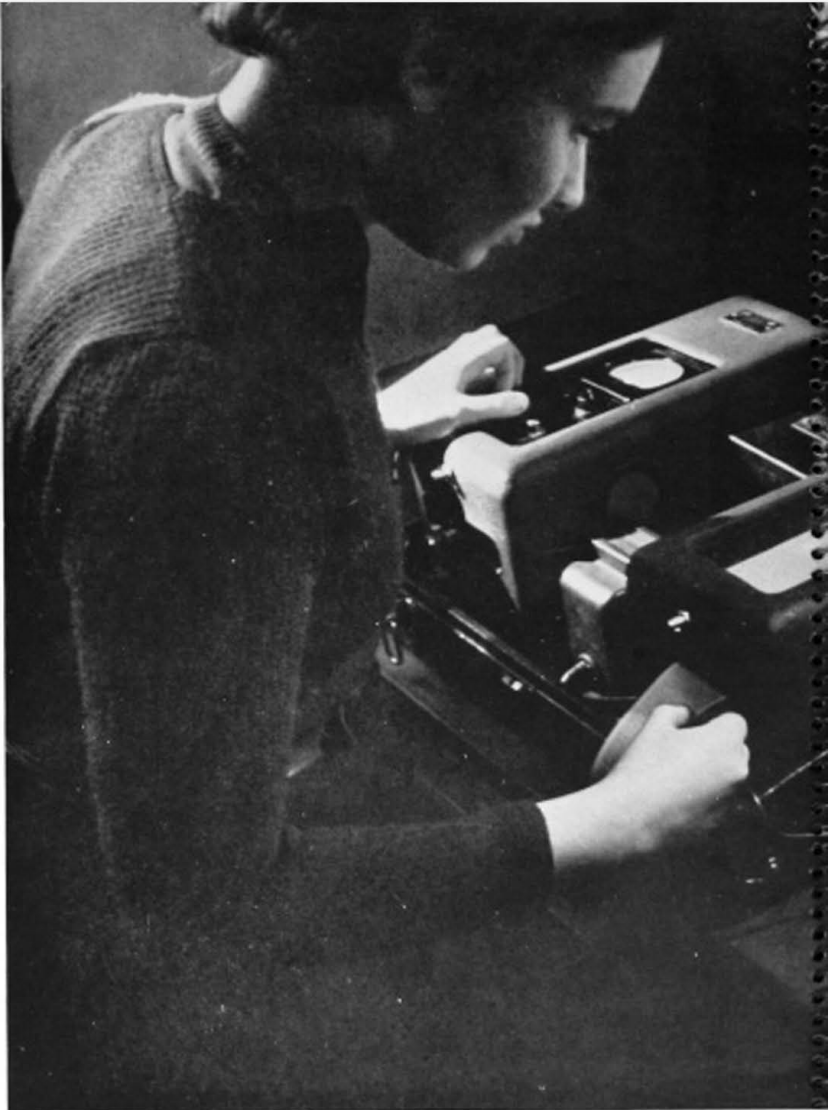
Electrically Measuring Surface Finish. Wear depends on quality of surface.
