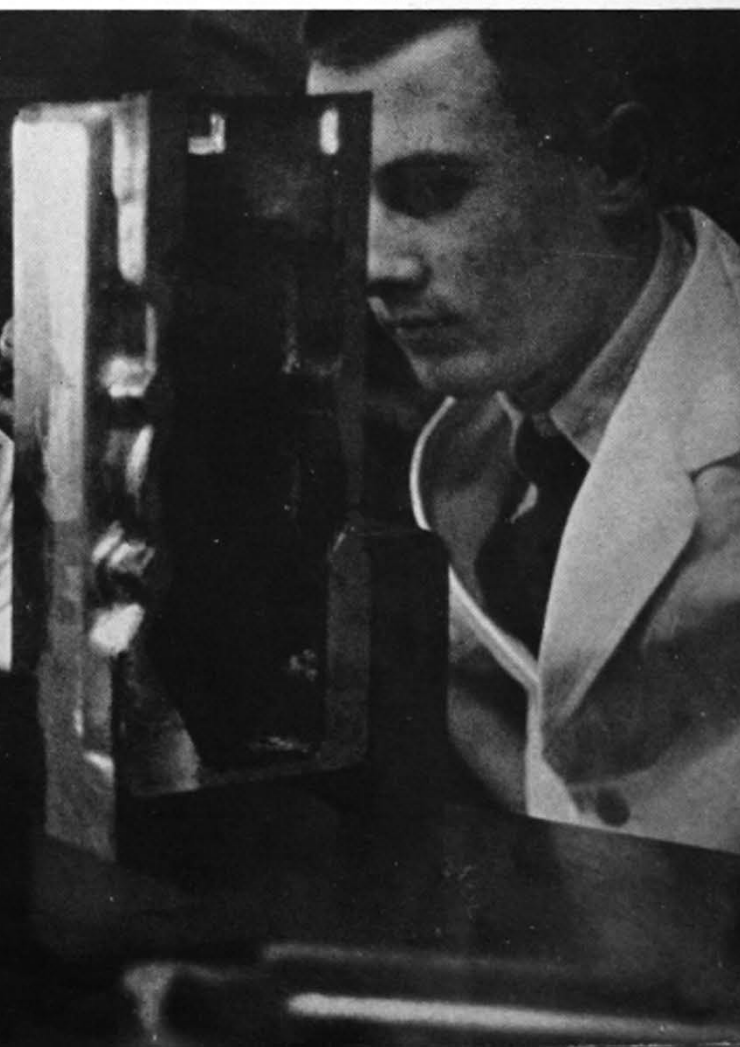
A case of extreme precision. Jig-boring in an air-conditioned, temperature-controlled room away from the noise and bustle of machine shops.
