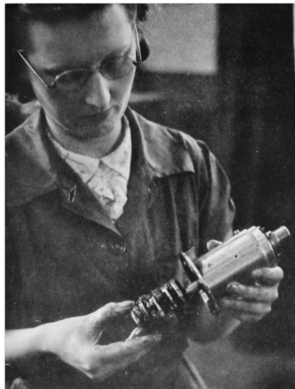
Component tests complete. The gear unit is heavily greased, for many years of trouble-free wear, and assembled.
